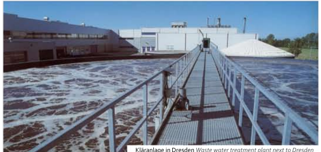
Kläranlage in Dresden Waste water treatment plant next to Dresden
