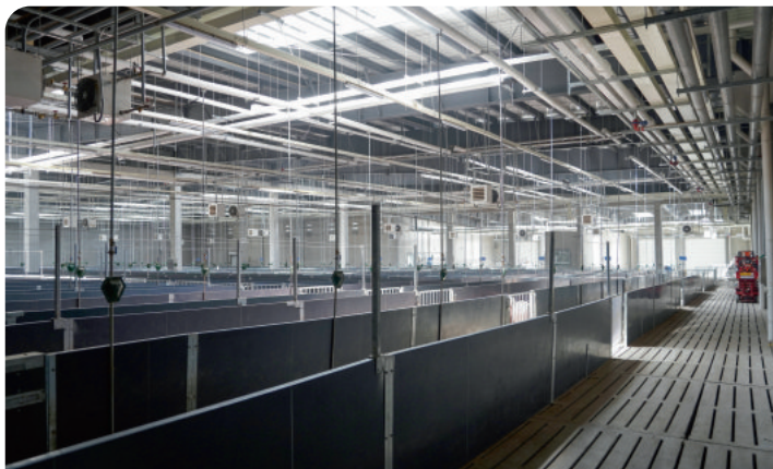
Animal welfare is gaining importance as an issue for the industry. Planning companies can make a major contribution to optimising the design of the enclosures and the race for stunning. Photo: Falkenstein
